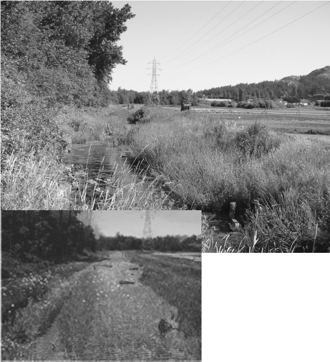
Blenkinsop Creek, Saanich BC. A completely new stream channel was built using the seventeen PFC processes and attributes as the design criteria. The stream was moved out of a ditch and restored to its functional condition.
