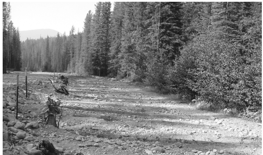
Mark Creek watershed, City of Kimberley (Aug 2003). The old road encroached on a small tributary to the drinking water supply (right) and prevented it from accessing its floodplain and dissipating energy. Logs were carefully levelled, spaced evenly across the old road bed and anchored with their root balls. The stream can now access its floodplain (old road) and the logs will slow the water, trap sediment and promote vegetation growth. A multiple-culvert array was installed in the new, elevated road to allow water to flow across the road without being concentrated and causing erosion downslope.
